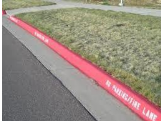
Figure 8 – Typical fire lane striping installation
